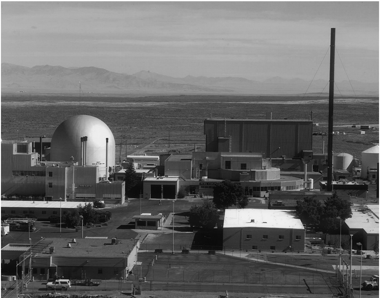
Fig. 1. The EBR-II reactor in the background with the power plant on the left and the fuel cycle hot cells on the right.
